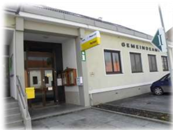
Figure 5. Location – PB3 municipality office. PS#1
