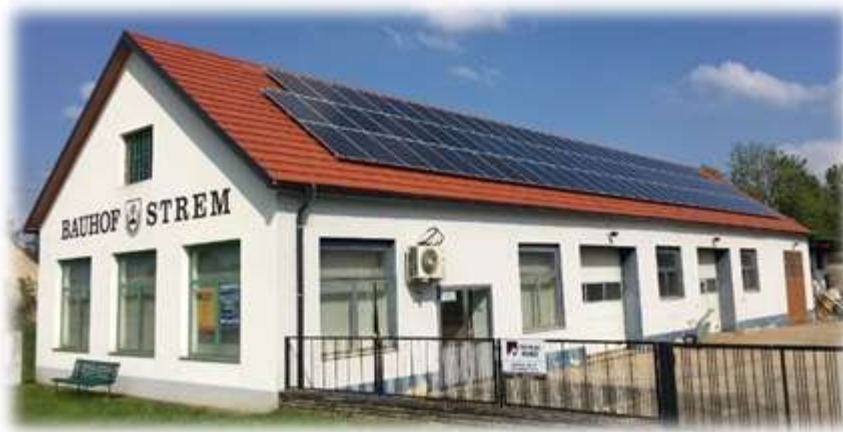
Figure 7. Location – PB5 machine hall. PS#1
