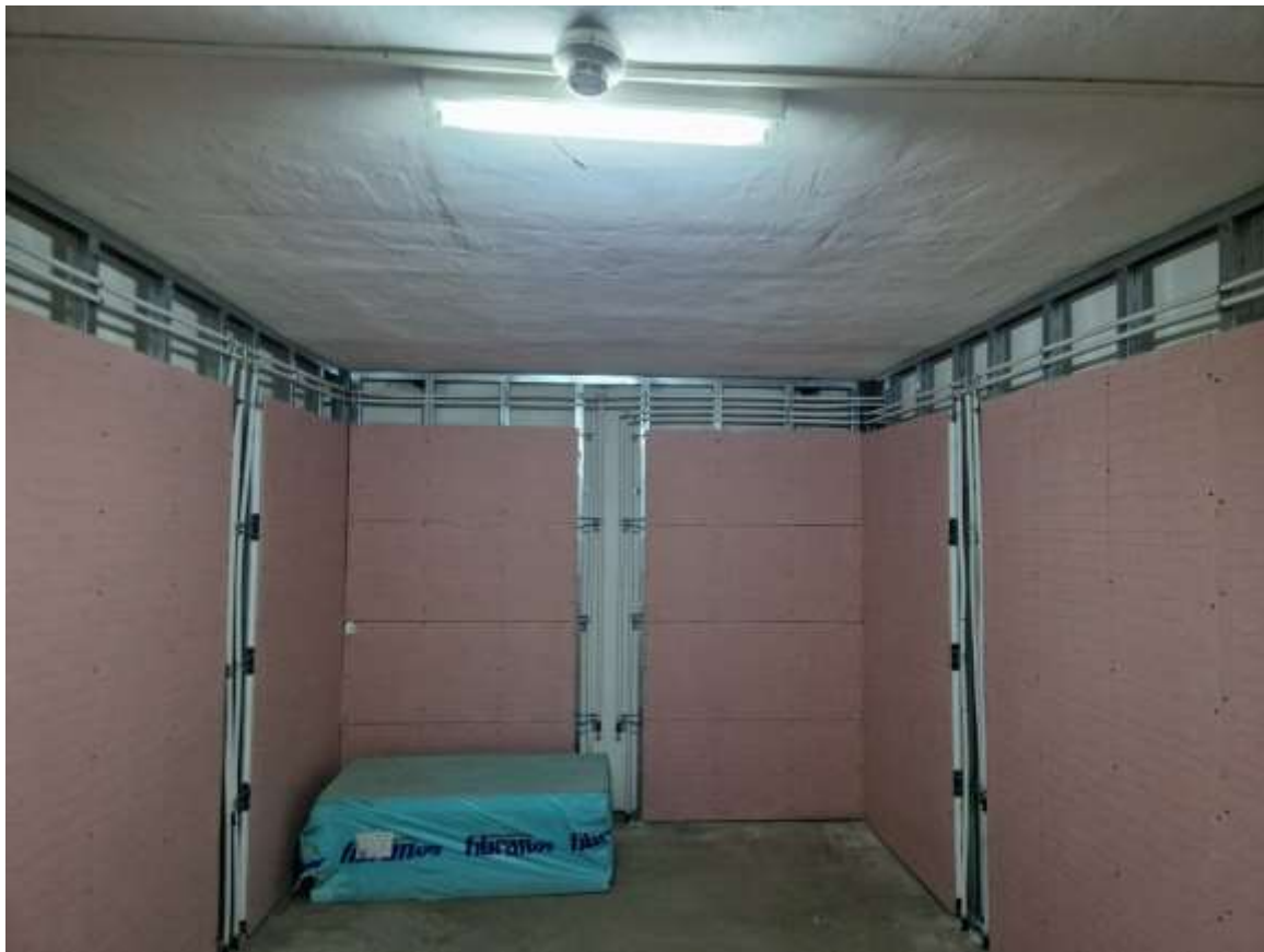
Figure 20. Interior GeoWall system
