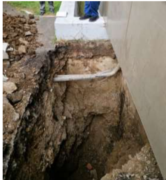
Figure 6. Execution of digging for measurements of the wall
