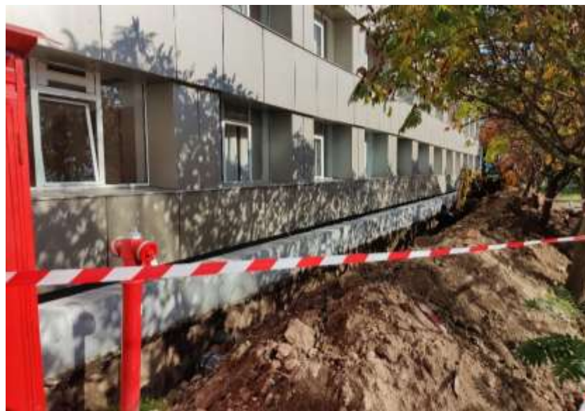
Figure 17. Excavations done for Evelixia exterior Wall
